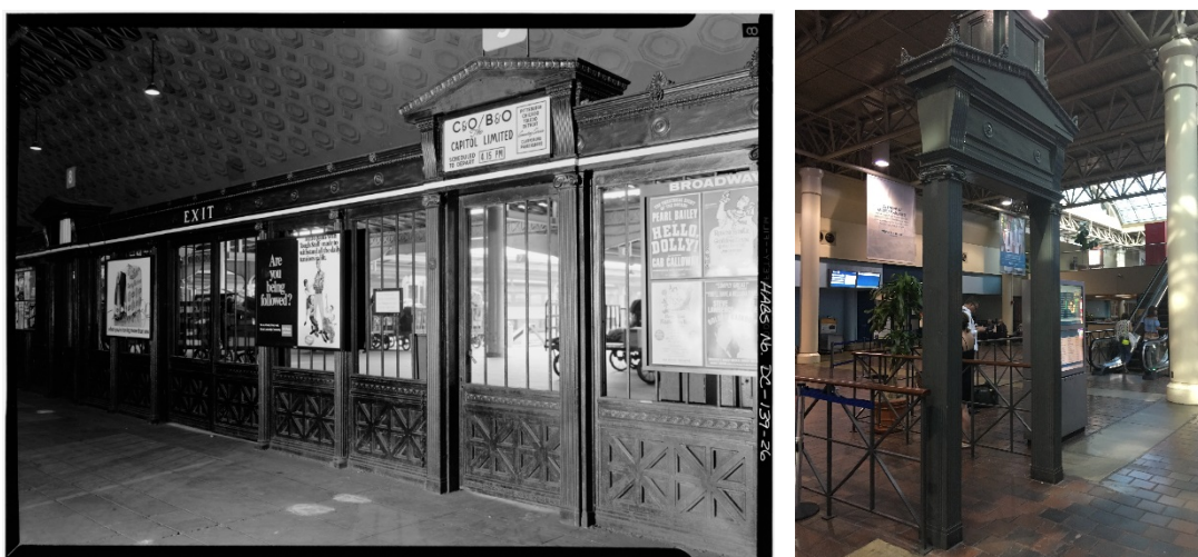
Figure 13. Historic Arches, Washington Union Station, 1968 and 2016
