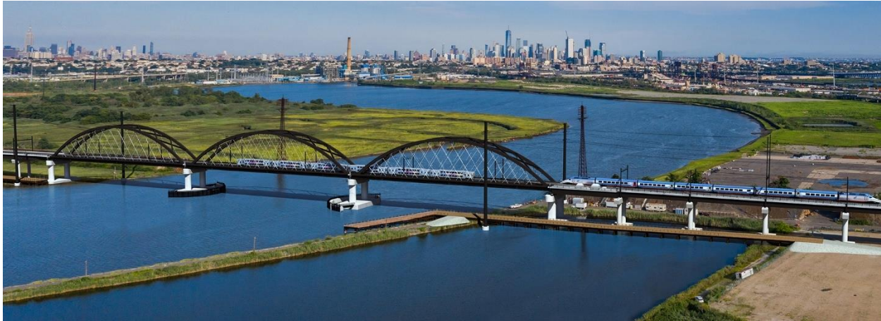
Figure 2. Future Portal North Bridge
