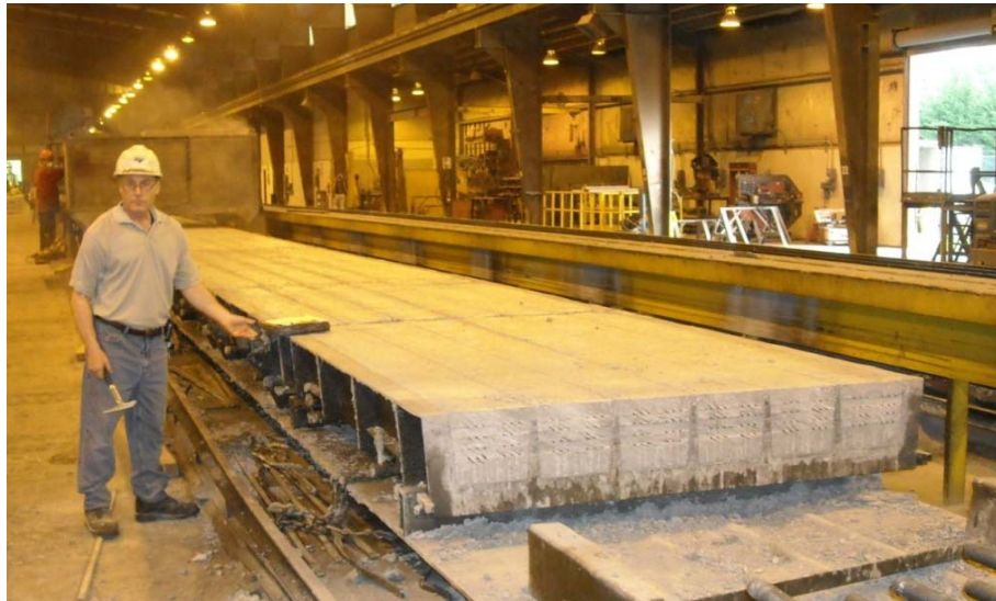
Figure 2: Amtrak Engineer Performing General Inspection of Concrete Ties During the Removal of Ties from Molds
